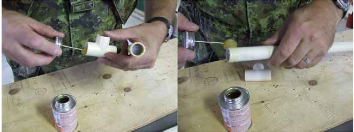
Figure 6-A Applying cleaner or glue to the joint surfaces before gluing.
